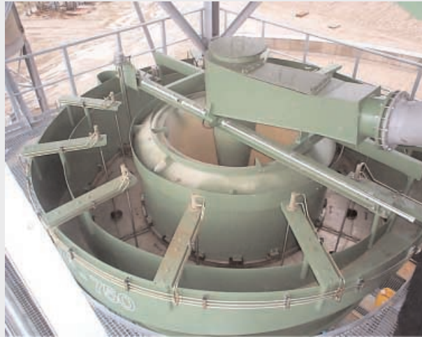
Fig. 8: allflux® during erection
